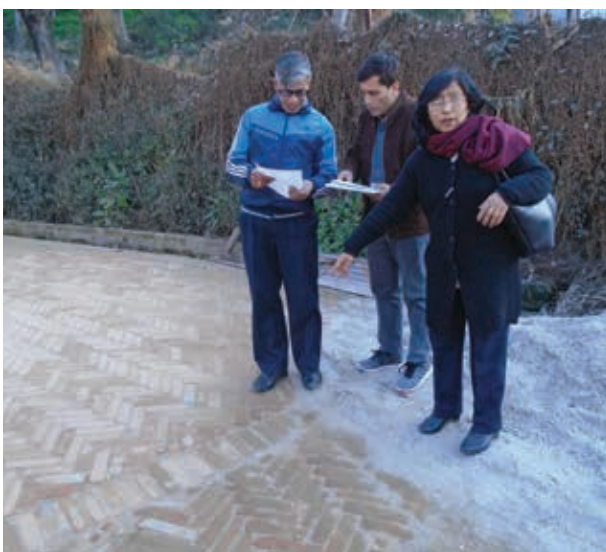
Monitoring of Brick soling work done by Bhaktapur municipality, Bhaktapur
