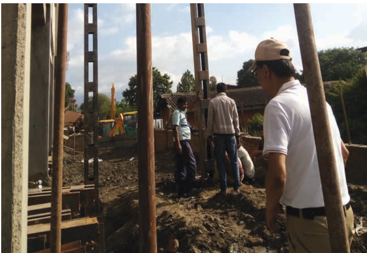
Columns for Fire escape
