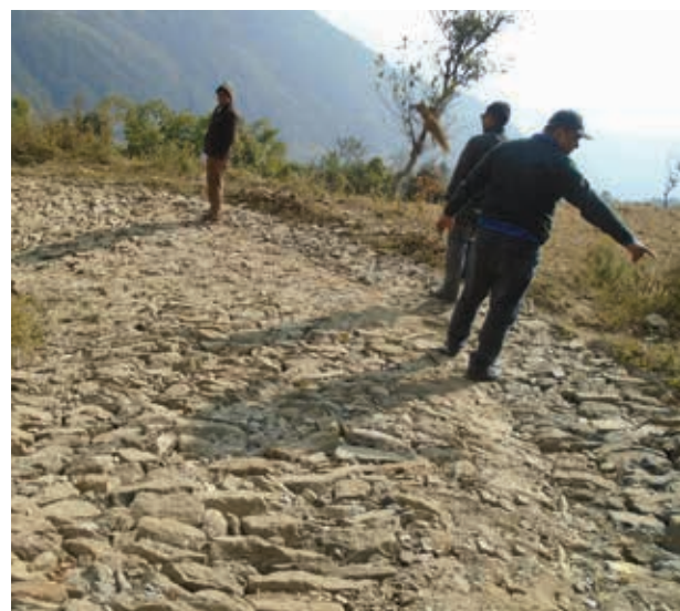
Observing dry stone soling work done by Rupakot - Majhuwagadhi Municipality, Khotang
