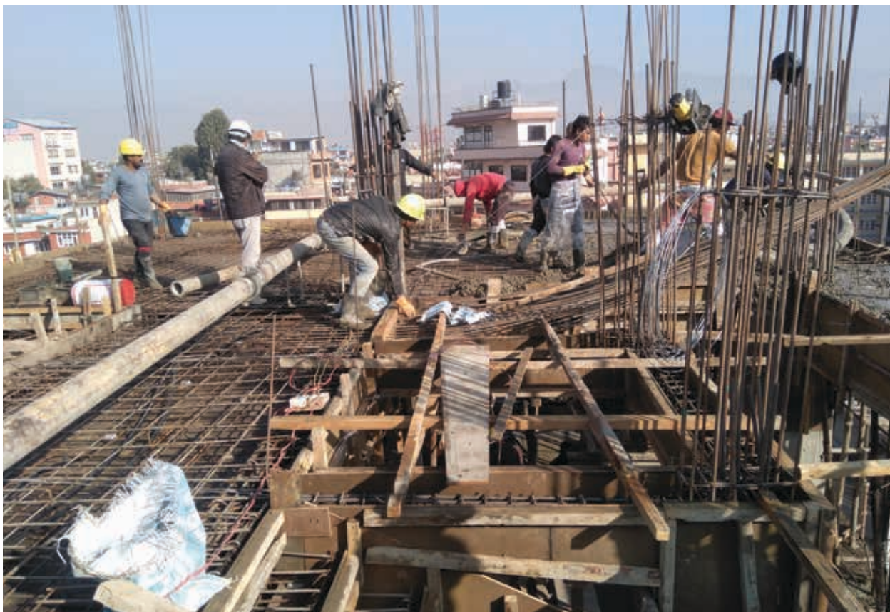
Over all building (North Elevation)
