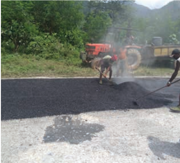
Road Maintenance work in progress
