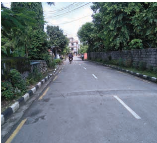
Road Maintenance work by Pokhara Sub metro
