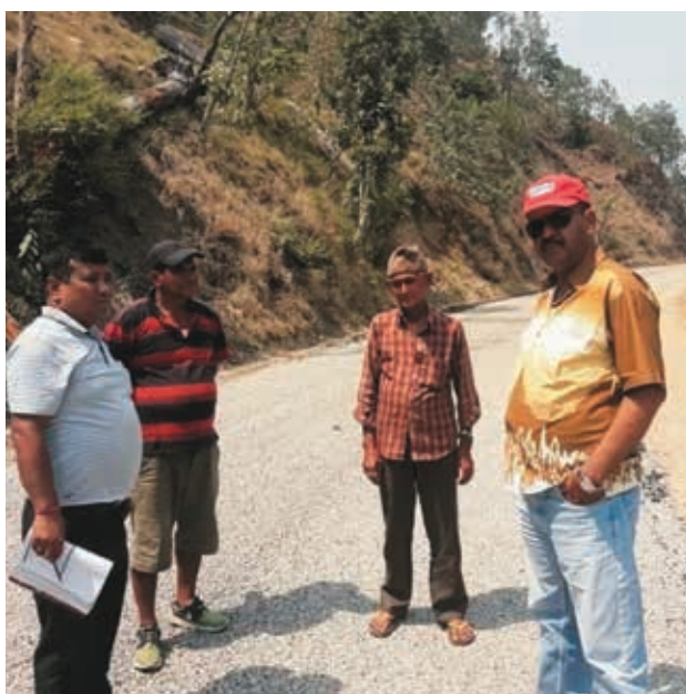
Re-sealing Work of Attariya-Dadeldhura Road Section monitored by Executive Committee Member
