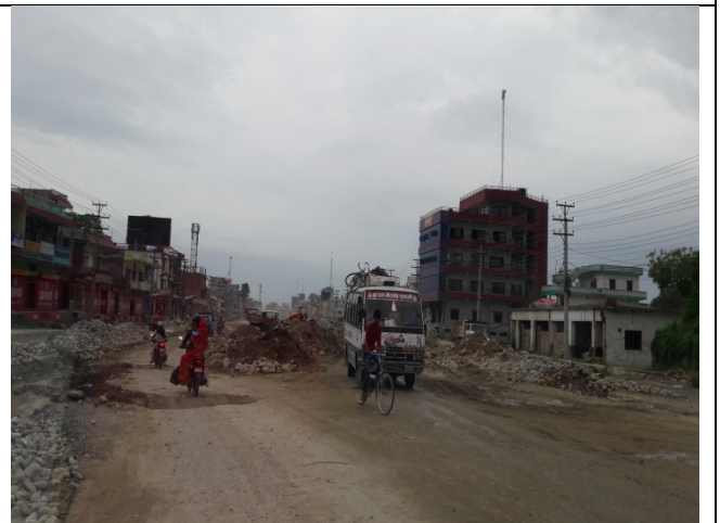
Condition of butwal bhairahawa road section
