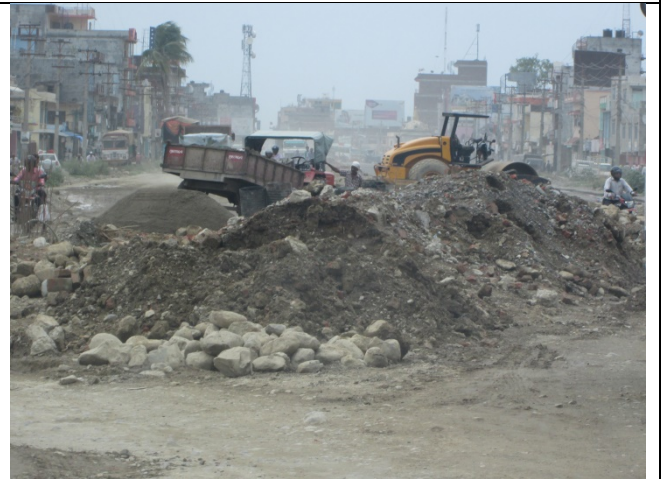
Butwal bhairahawa road under construction
