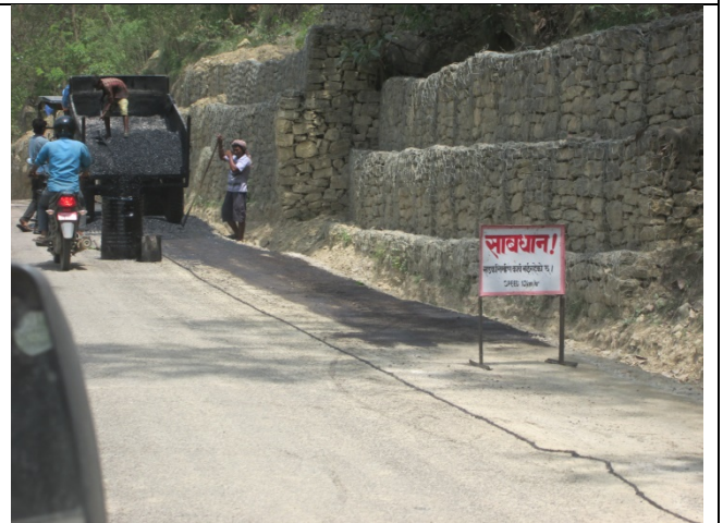
On going repair work (Chhinchu-surkhet section)
