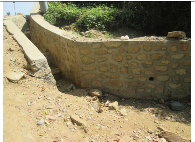
Dadekdhura – Bagarkot Road section, which is under construction
