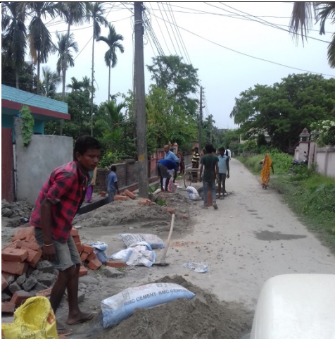
Drainage Construction Biratnagar
