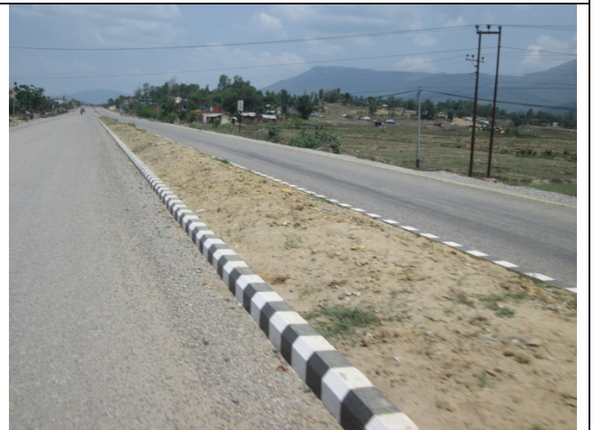
A newly constructed road with median at Birendranagar, Surkhet
