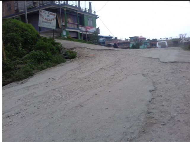
Junction of Hile-Bhojpur road
