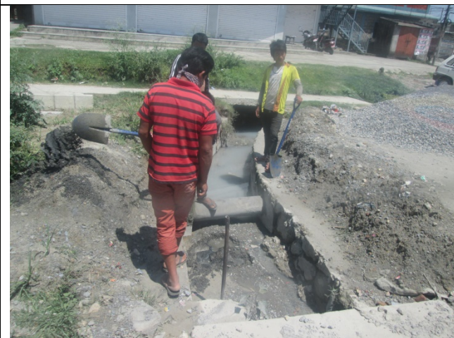
Cleaning the side drain on Pokhara Baglung road
