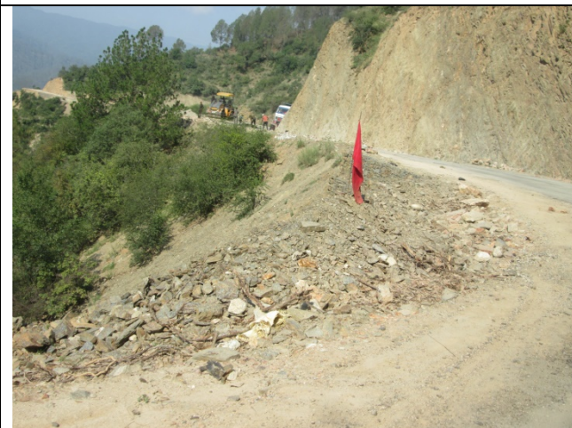
Dadeldhura – Bagarkot road under construction
