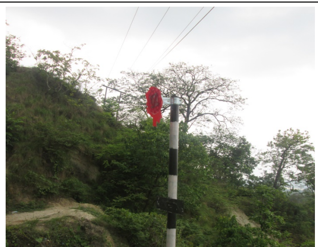
Theft of the mirror, which was kept on side of the road to reduce road accident.
