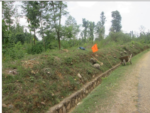
A view of continuing routine maintenance work
