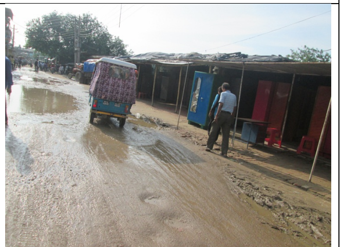
Muddy road condition along Thori-Sirsiya road
