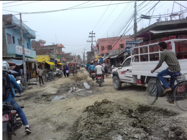
Condition of Road on the way to Snatiban & Bigyan Kendra (Biratnagar)
