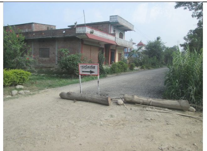
A temporary diversion at Taulihawa road
