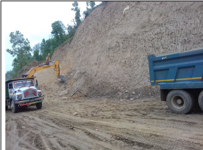
On going construction work, Galchhi-Trisuli Road
