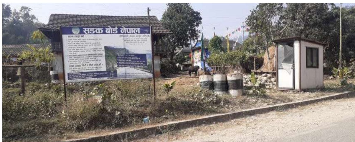
Photo No. 7. Temporary Shed for Toll Collection
