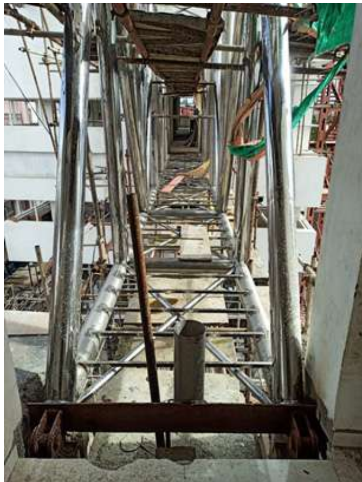
Photo No. 4. Erection of Truss Bridge in Progress
