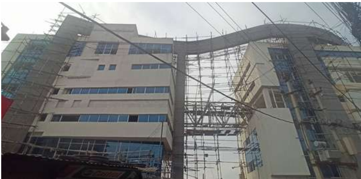
Photo No. 1. North East Elevation of Building
