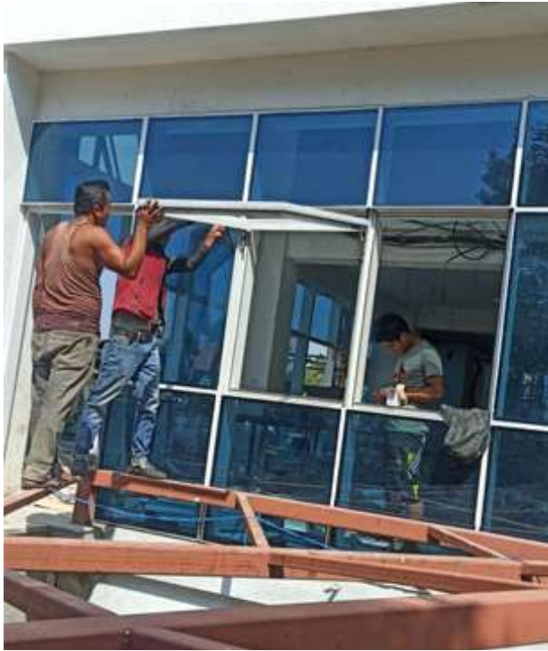
Photo No. 2. Glazing in Progress
