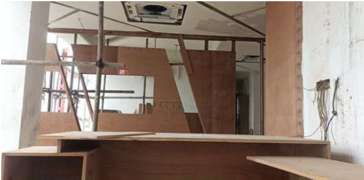
Photo No. 5. Partition Works in Progress
