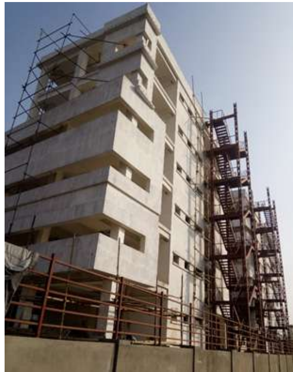
Photo No. 3. Fire Escape
