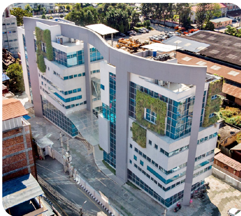
Photograph No. (2) RBN Building (North-East Elevation)
