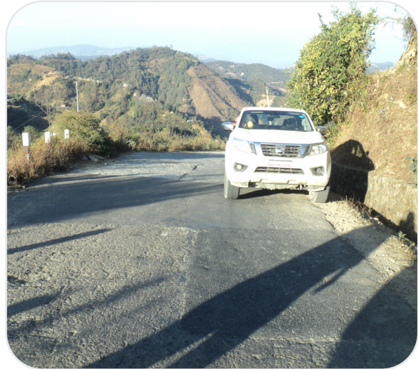
Photograph No. (12) Field Monitoring at Bethan Chwok RMU
